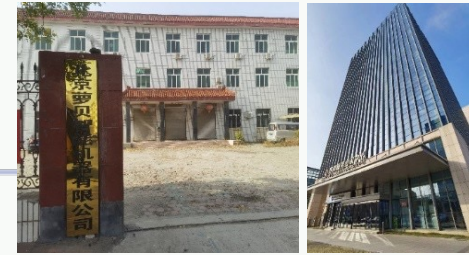
Beijing LOBO Factory
